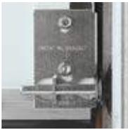
Helps prevent serious injury that could occur if the bottom bracket were removed with the garage door closed and under tension.
